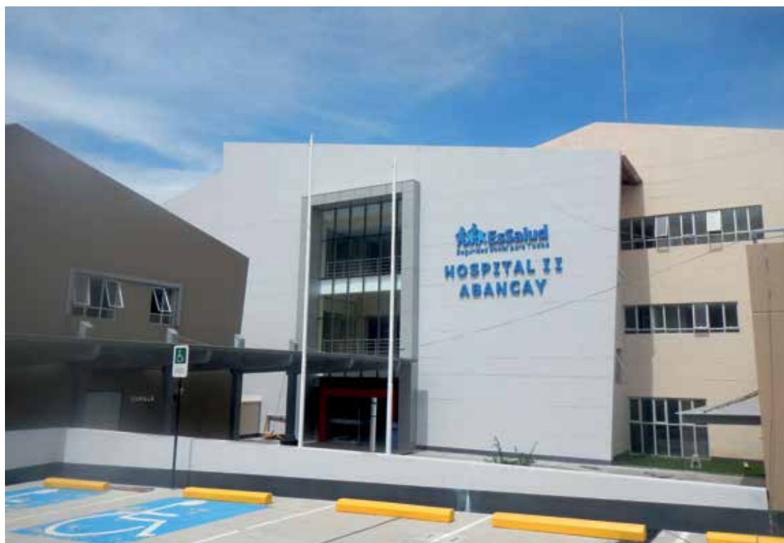
➤ Hospital II de Abancay.
